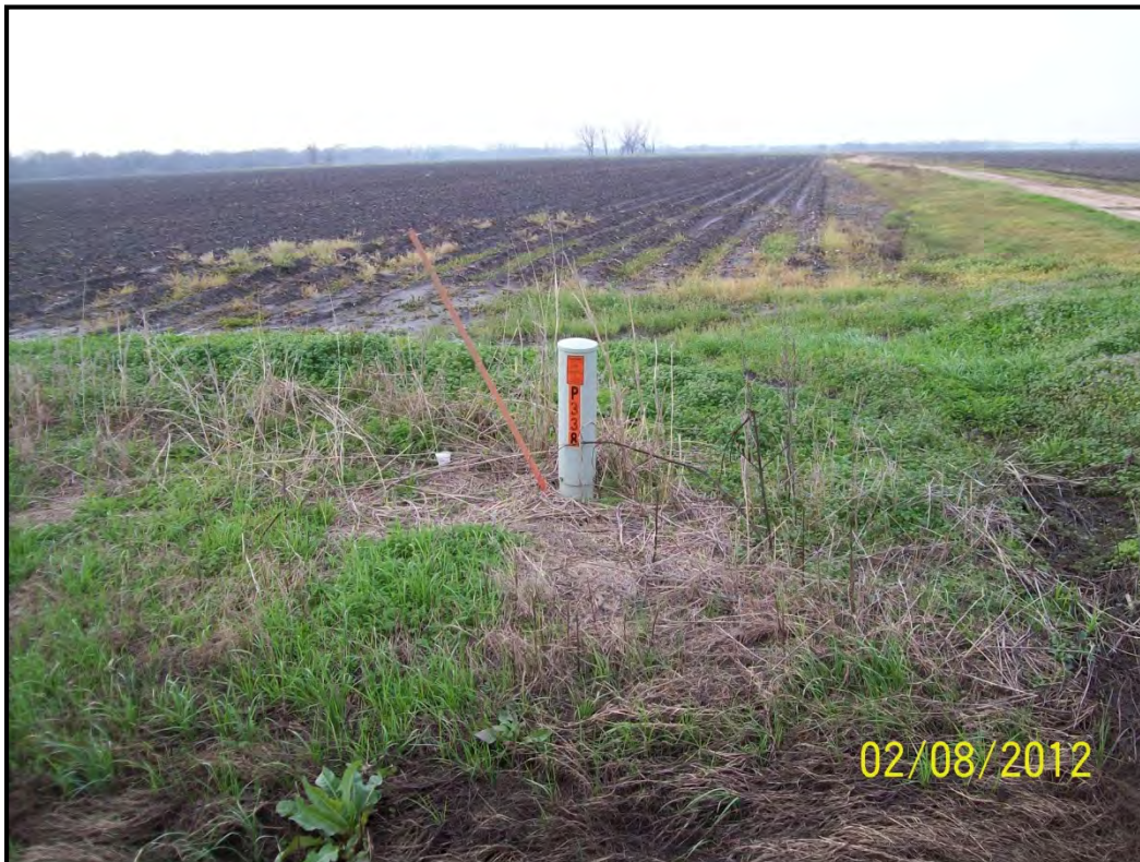
Photograph 8 – Looking south, view of an AT&T underground telephone cable marker located on the northern Property boundary.
