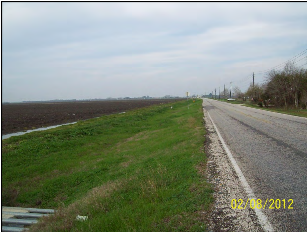
Photograph 2 - Looking west, view of the northern Property boundary along F.M. 1161.
