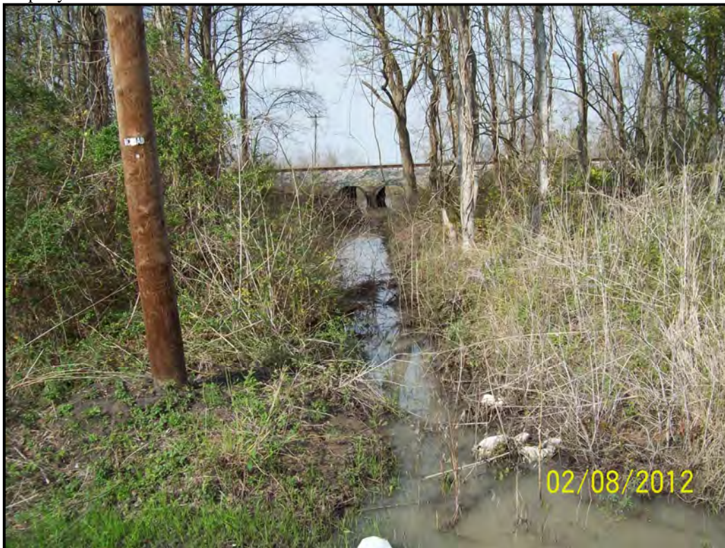
Photograph 18 – Looking west, view of water draining from the Property under the Southern Pacific rail lines located along the eastern Property boundary.
