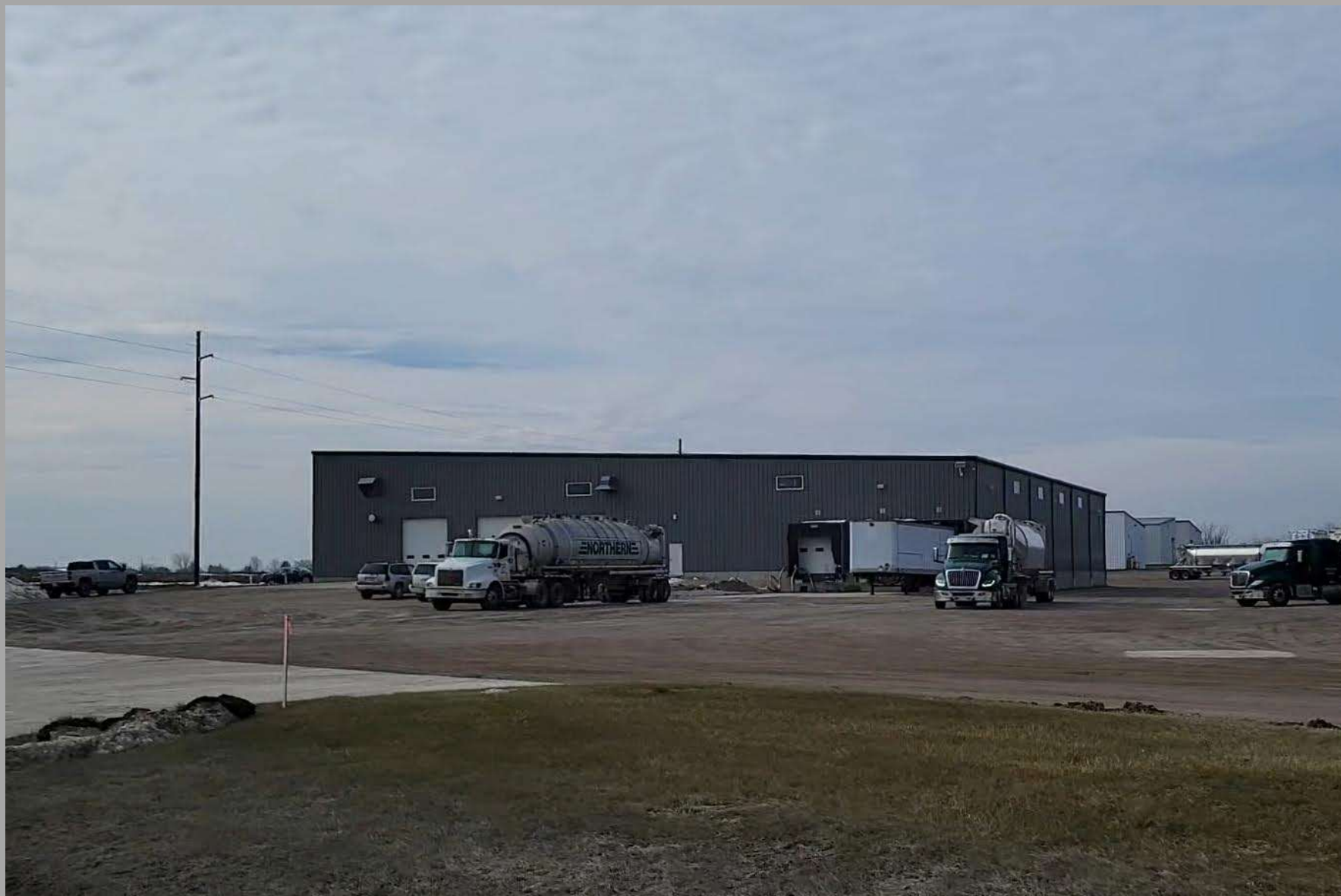
Photo 6 – 605 Industrial Drive – Facing Southwest, looking at North and East elevations
