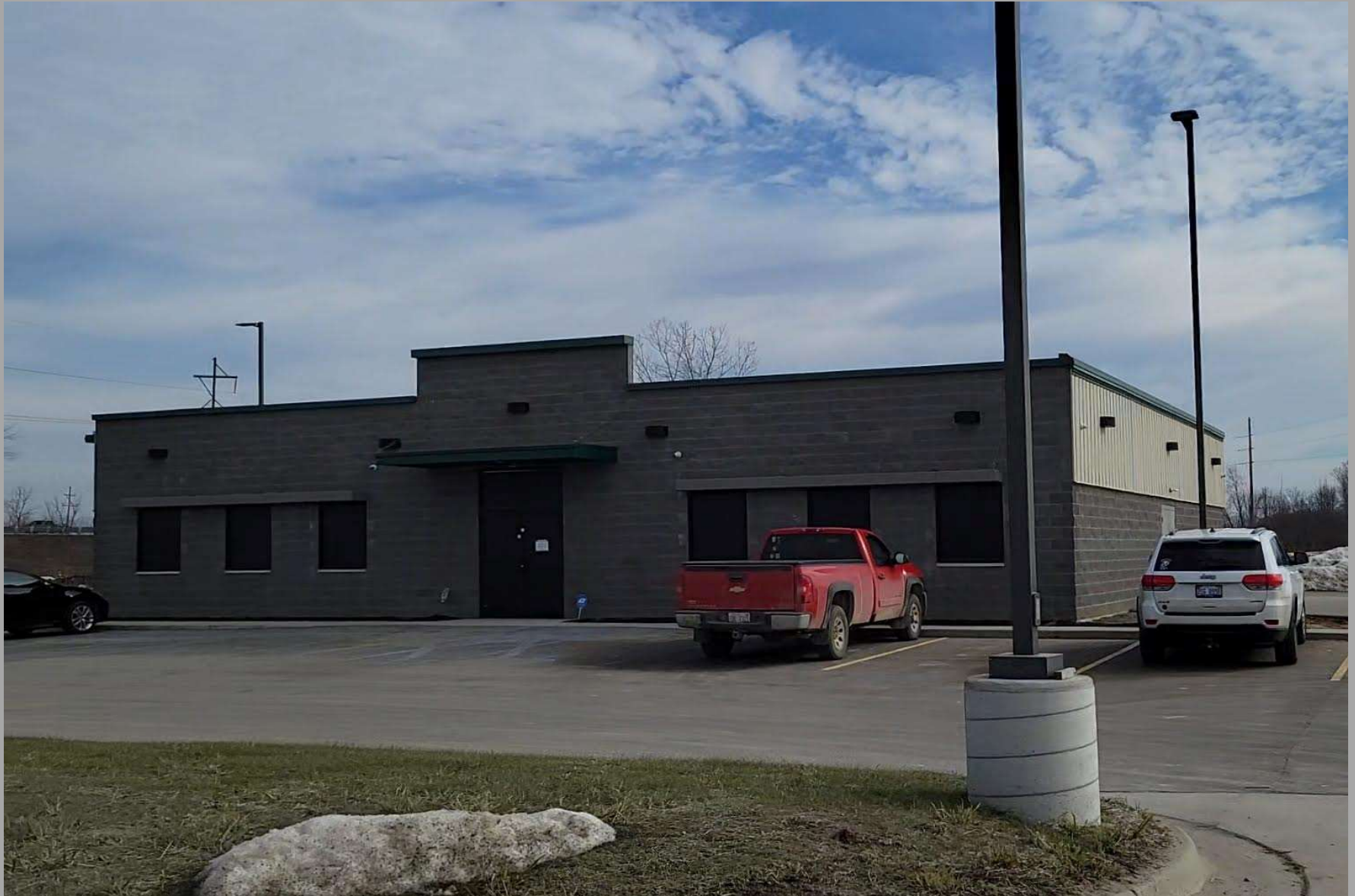
Photo 7 – 690 Industrial Drive – Facing NorthEast, looking at South and West elevations
