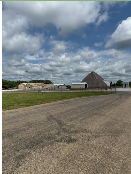
View of storage area located at Highway Department facilities on southern adjoining property
