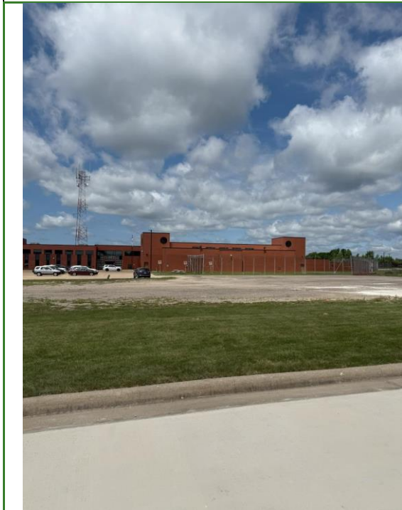
View of southern adjoining property, facing west
