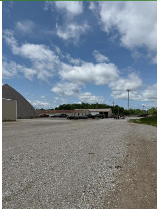
View of southern adjoining property facilities at Highway Department
