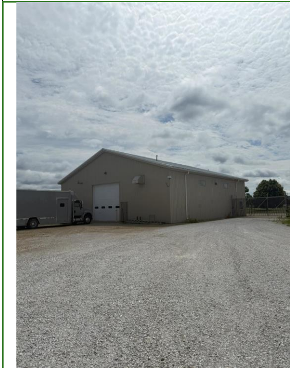
View of structure from the impound lot facing east
